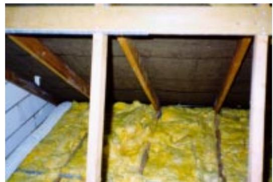
Insulation packed into the eaves has blocked ventilation paths. When the insulation quilt was lifted it was saturated with water condensate
