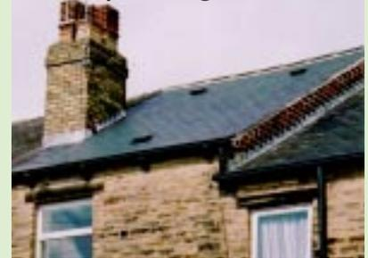
Never fit ridge or high level vents as the only means of ventilation — they must always be used in conjunction with vents at or near eaves level. With high level vents alone, the air flow over the ridge creates a pressure drop inside the roof space, which sucks moist air from the house into the roof.
