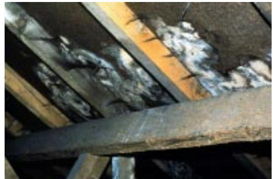
Condensation in the roof space can lead to mould growth and rot in the timbers
